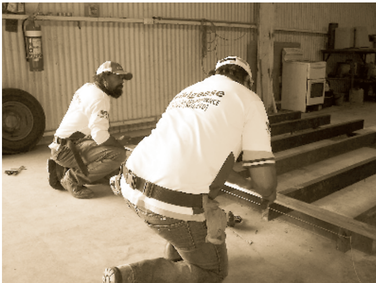
Apprentices Arnold McGrady and Leon McGrady setting out timber floor joists for the Stage 3 Boggabilla/Toomelah Project, run by the Batchelor Institute of Indigenous Tertiary Education.
